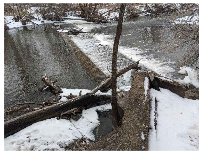
2 EXISTING CONCRETE WEIR & RIVER RIGHT EMBANKMENT
