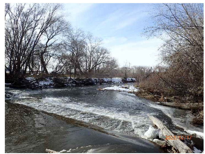
5 EXISTING CONCRETE WEIR AND RIVER LEFT BANK VIEW
