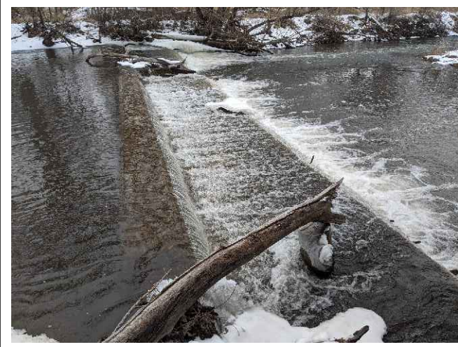
1 EXISTING CONCRETE WEIR
