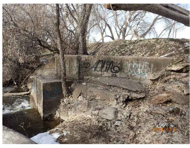
3 RIVER RIGHT CONCRETE EMBANKMENT (DETAIL)
