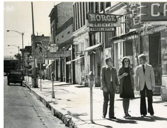
By the 1970s, street trees had all but disappeared from 25th Street. The lack of human comfort contributed to the hostile pedestrian experience already created through Urban Renewal programs in the middle of the century that saw businesses and residents relocate to the suburbs.
